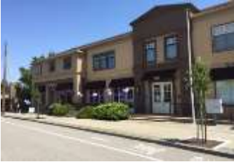
Umpqua Bank Building (999 Grant)
