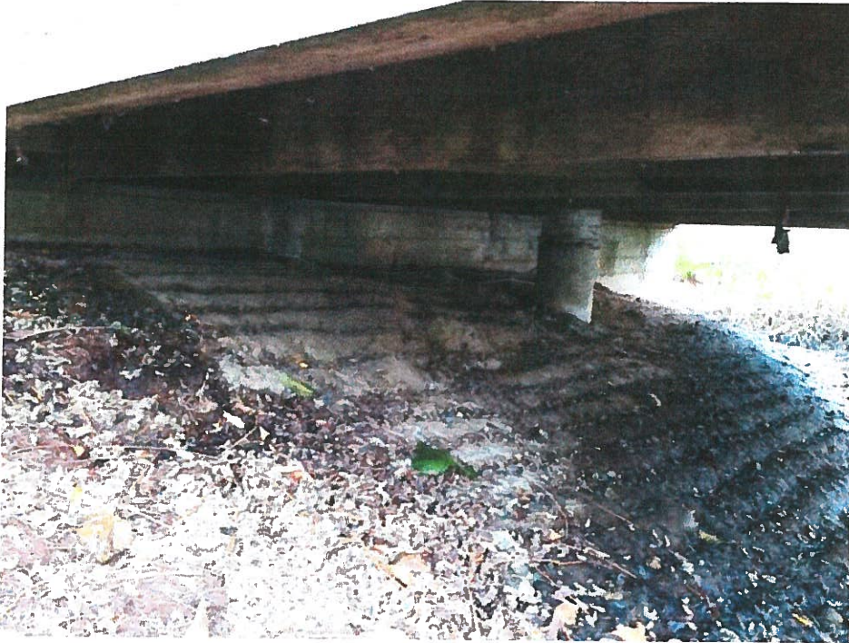
Foundation View taken 6/1/2015
